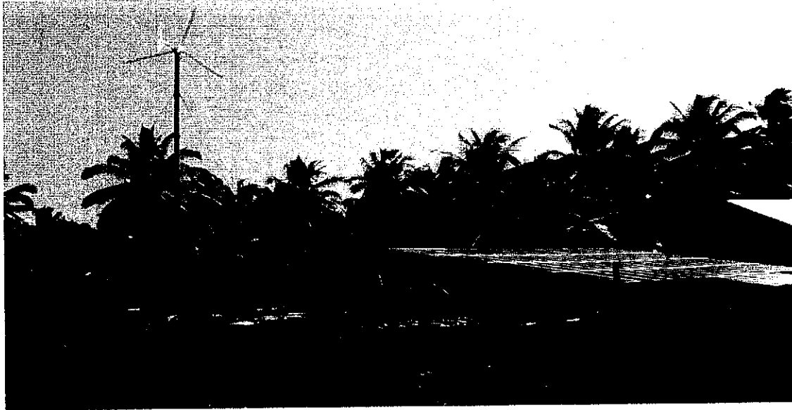
Outside view of the Hybrid PV-Wind Turbine System
